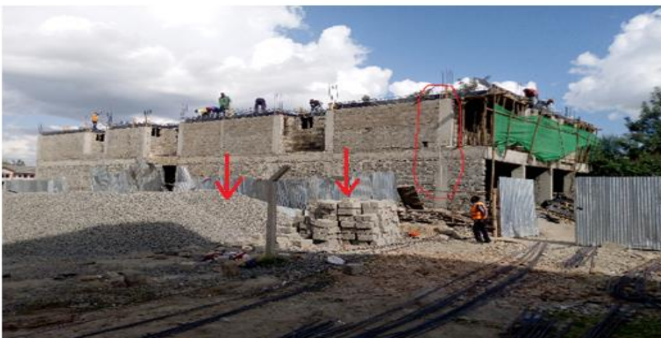
Figure 6: Material delivery to construction area
