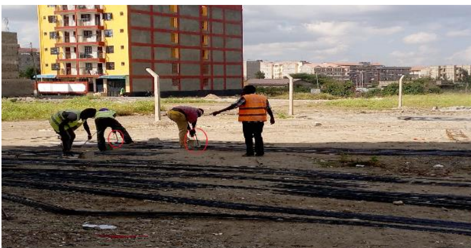
Figure 7: Cutting reinforcement steel using hand tools.
